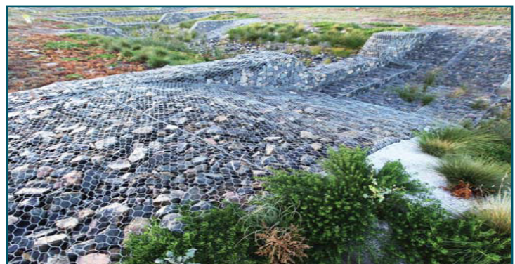
Typical Castoro Reno Mattress Application
