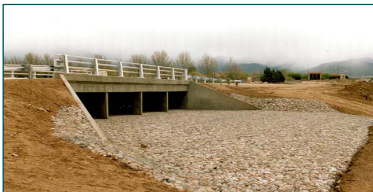
Typical Castoro Reno Mattress Application
