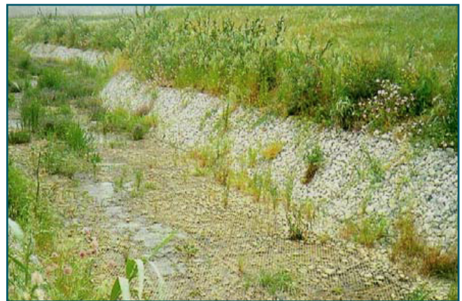
Typical Castoro Reno Mattress Application
