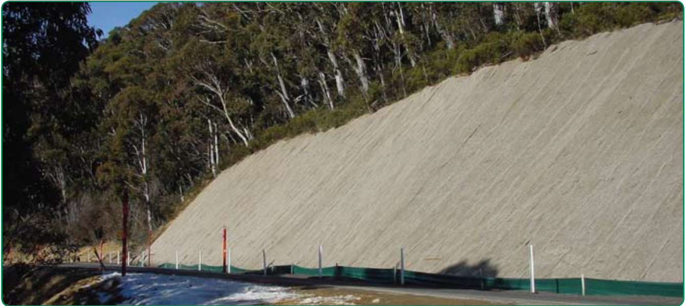
Jutemat steep slope erosion protection
