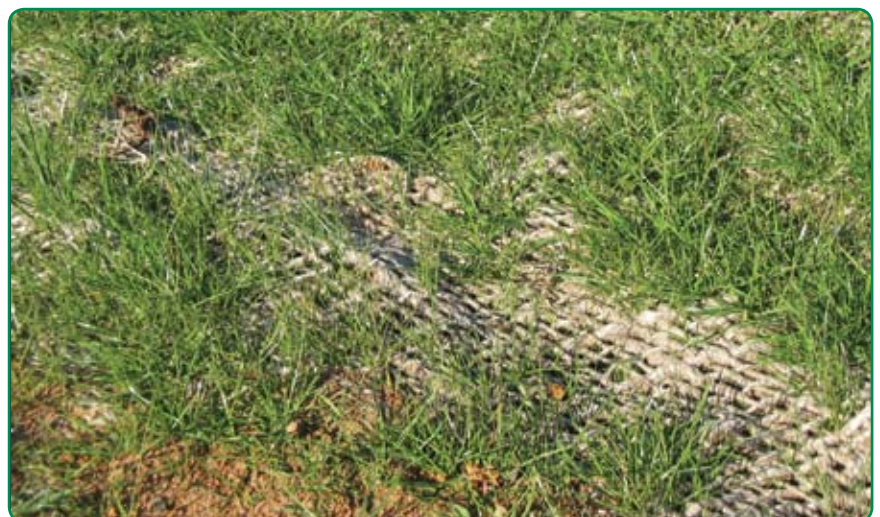
Jutemesh allowing vegetation growth
