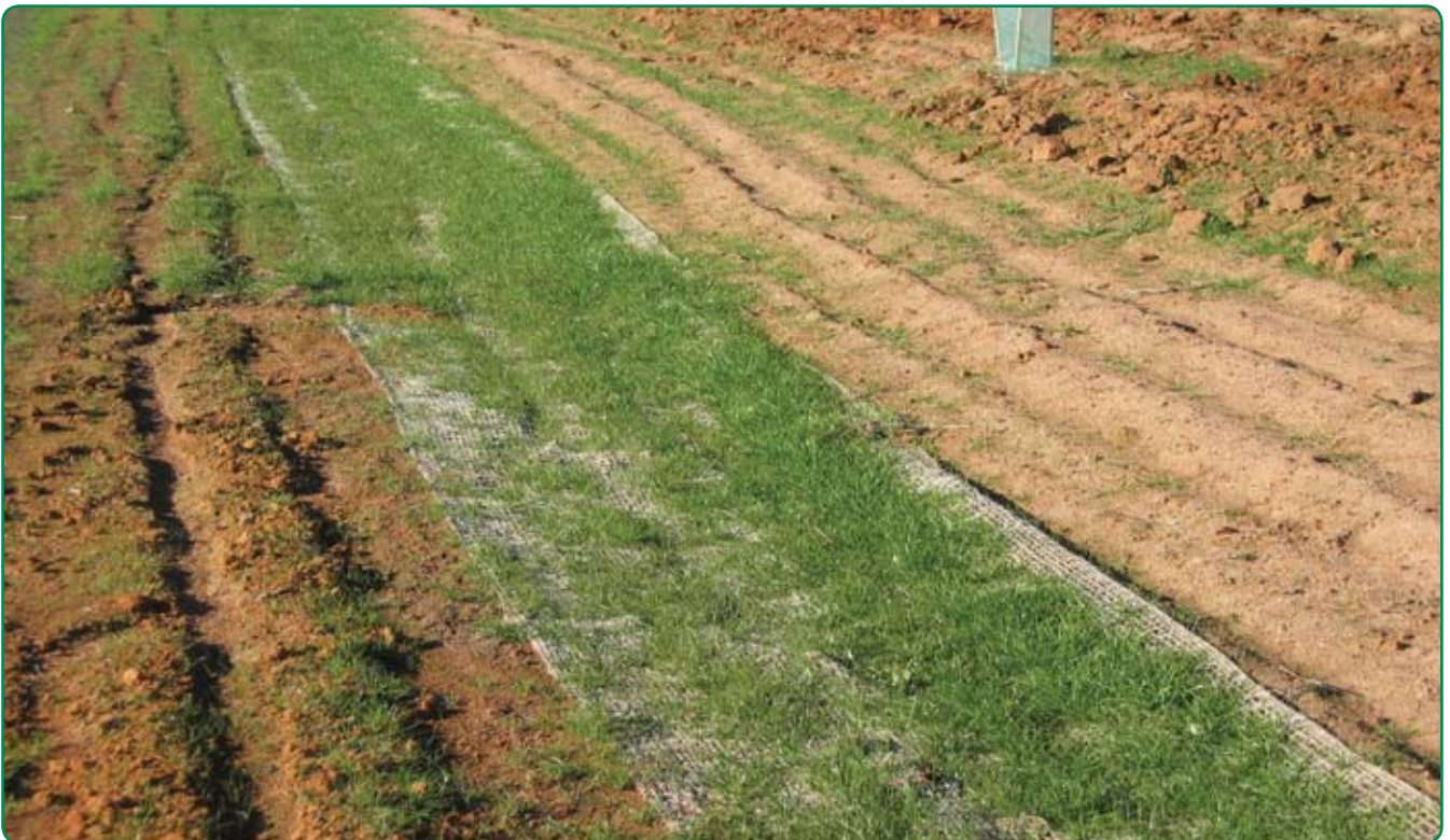
Jutemesh swale drain
