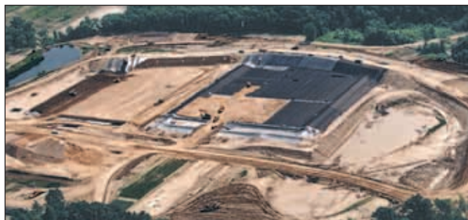
A double lined, multi-cell landfill.
