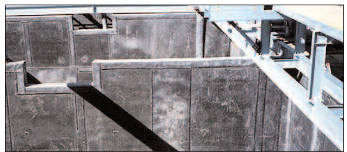
HDPE liner deployed over concrete in a wastewater treatment aerobic digester.
